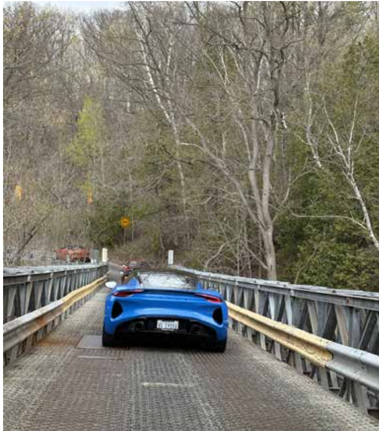
ABOVE Chris Marson's Emira on one lane-two way bridge.
